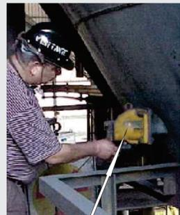
The source housing of a level gauge incorporating a gamma source. The detector is on the opposite side of the vessel.
