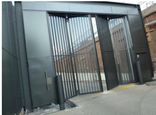
FIG. 43. Hardened steel grated door (may be guarded or unguarded).
