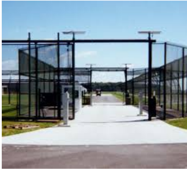
FIG. 20. Example of a vehicle access control portal.
