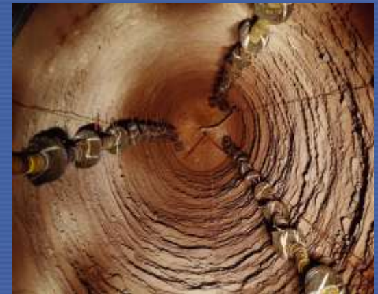
Interior view of borehole
