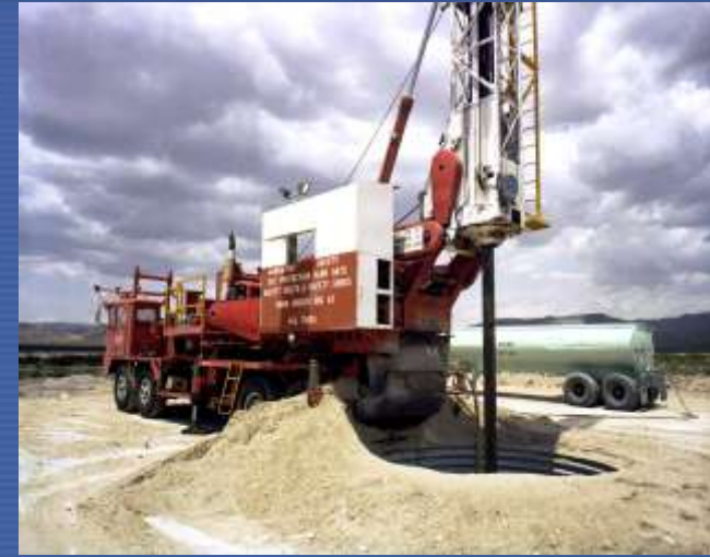
Drilling a Large Diameter Borehole with a Corrugated Metal Surface Casing
