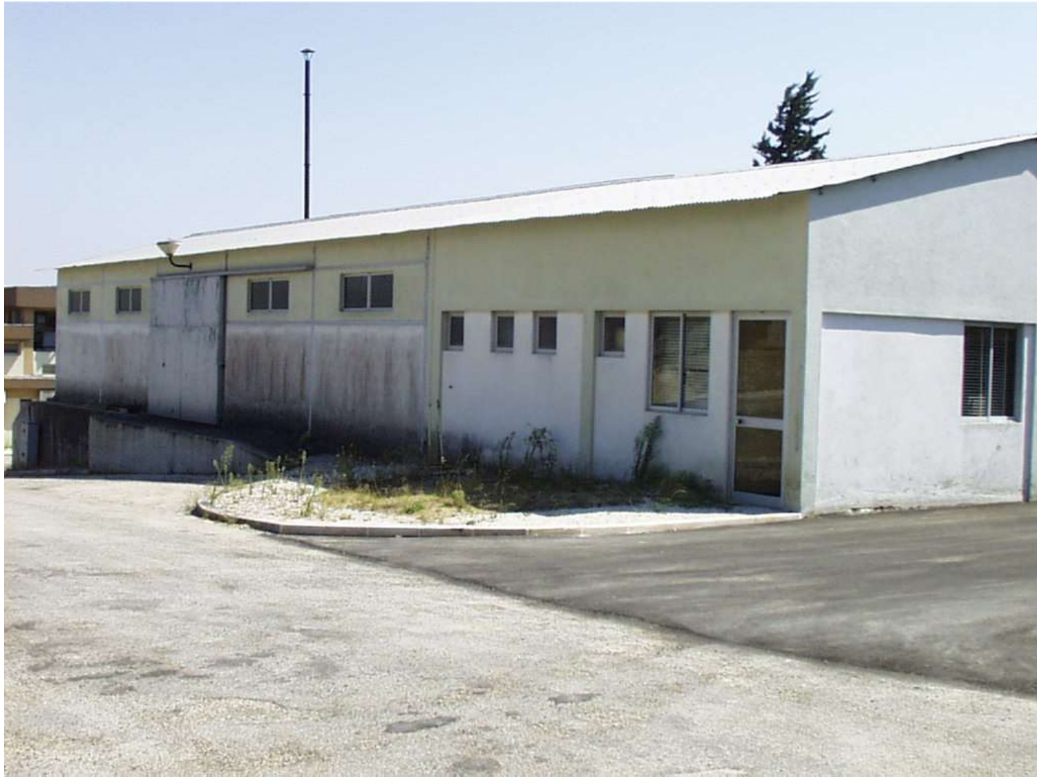
ITN, Radioactive Waste Interim Storage Facility (PAIRR)
