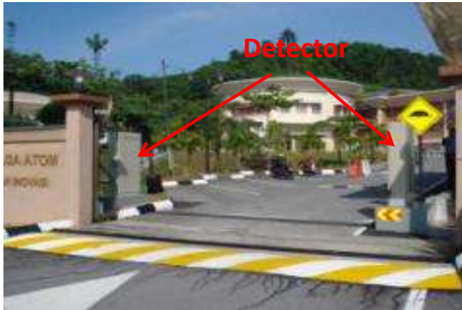
Alarm triggered at AELB entrance
