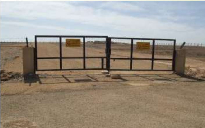
Partially Constructed processing building at Sewaqa
