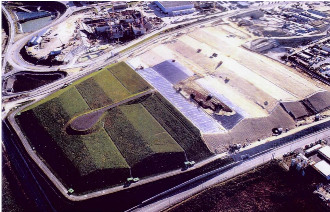
Figure 5.3 1993 aerial view of the cap being constructed over the Centre de la Manche LLW disposal facility in France.
