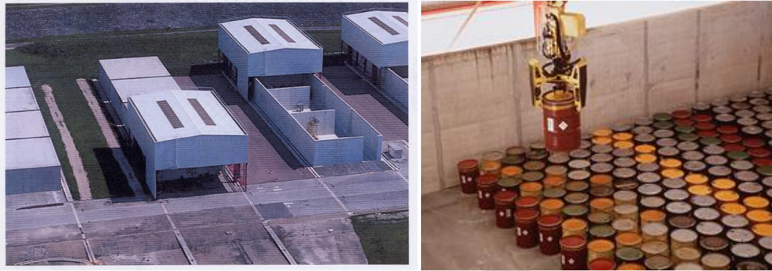
Figure 5.2 Waste trench and manual disposal practices at the Centre de la Manche disposal facility (top) and improved facilities and disposal practices at the more modern Centre de l'Aube disposal facility (bottom) (Tichauer 2010).
