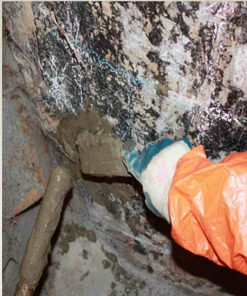
Plugging of bored holes
