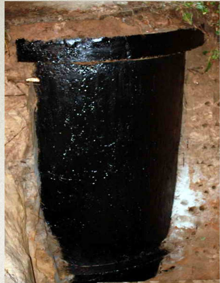
Renewal of insulation
