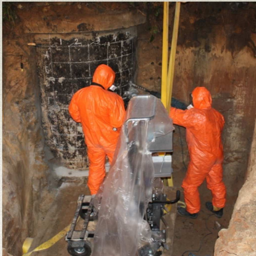
Drilling of holes
