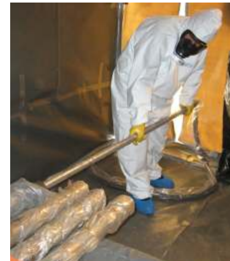
Sandblasting of tubings
