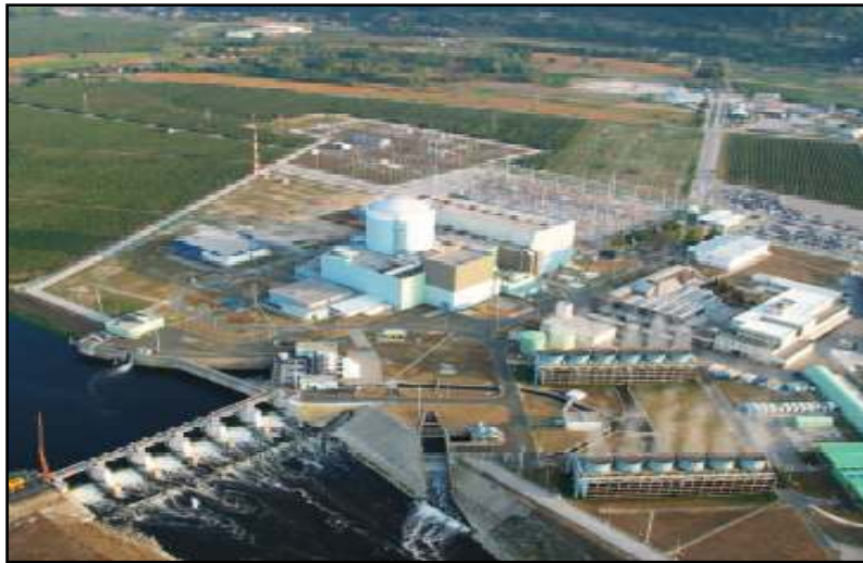
1. Krško Nuclear Power Plant
