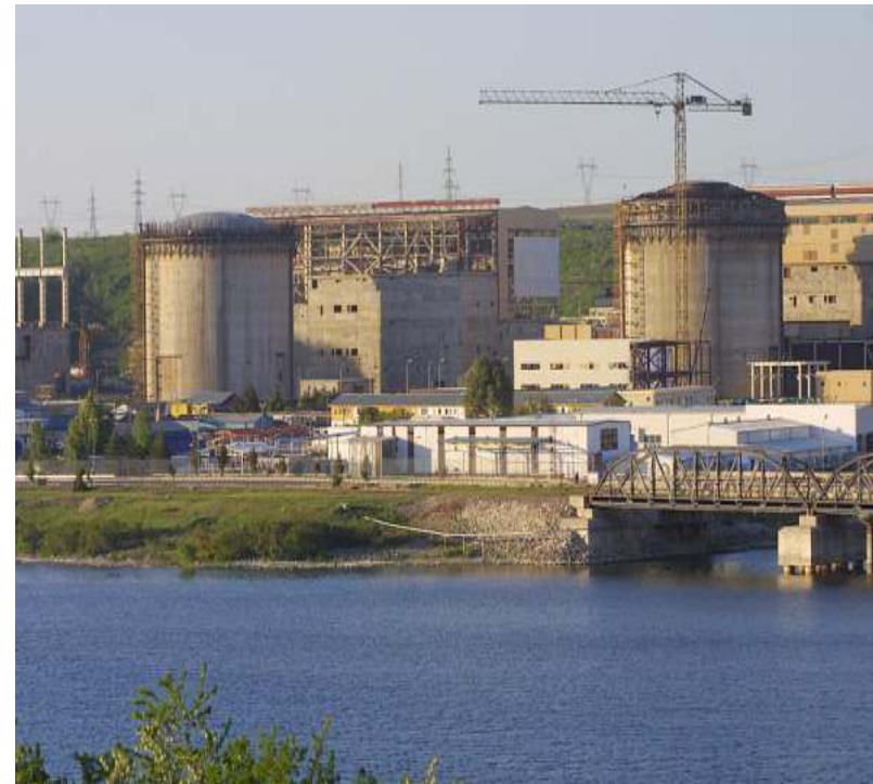
Energonuclear S.A. Units 3 & 4
