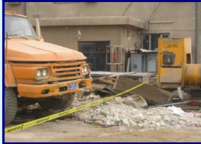
Site preparation and fencing
