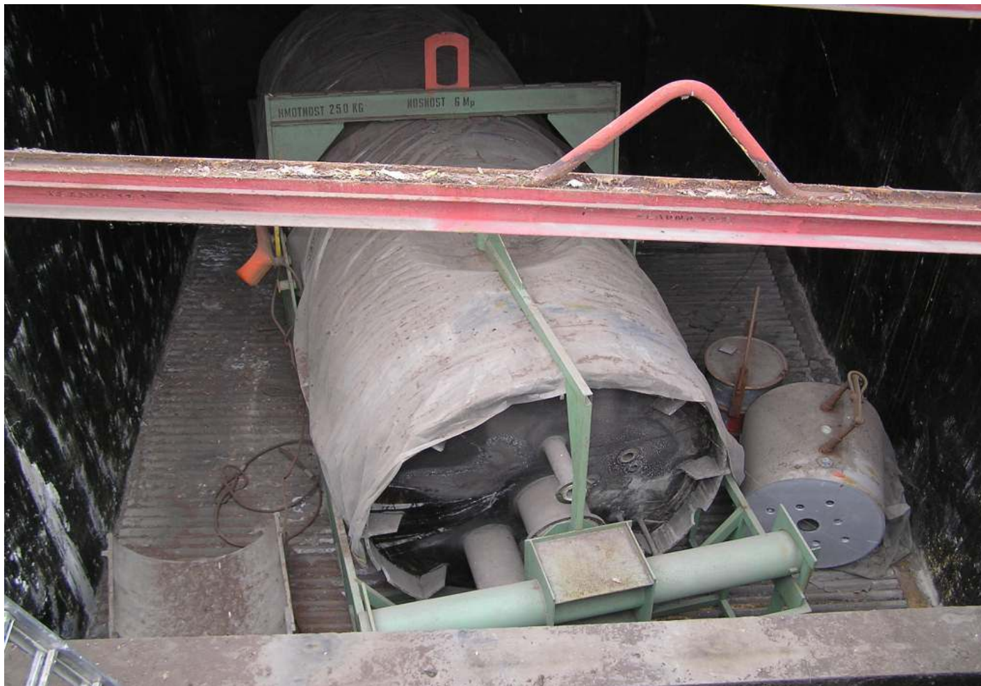
Stored RAW – VVR-S research reactor vessel
