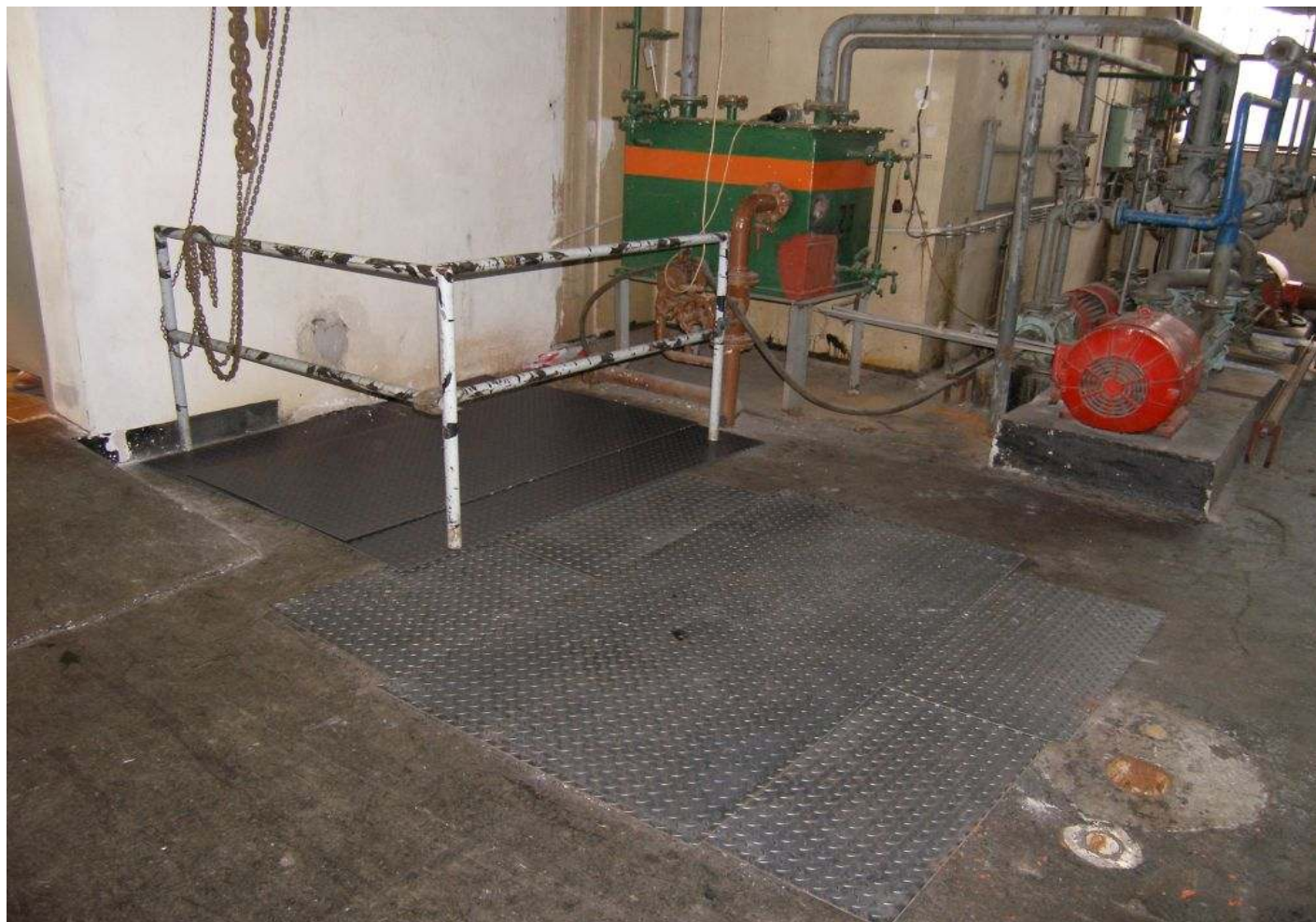
After evaporator decommissioning
