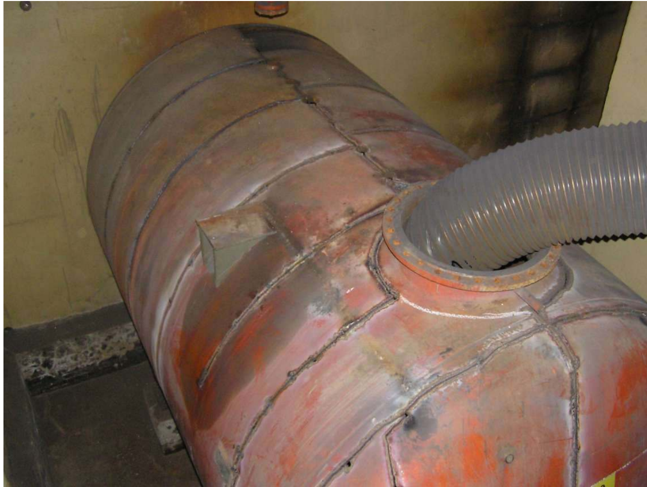
Storage tank during segmentation
