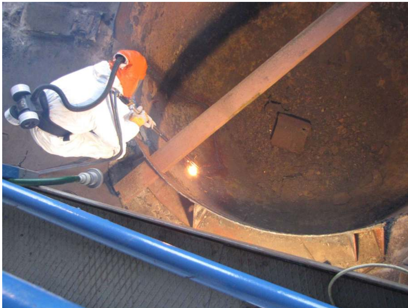
Segmentation of sedimentation tank
