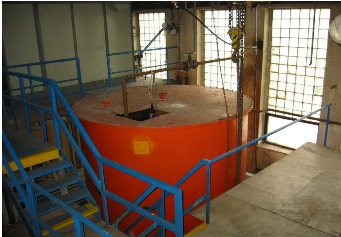
Sedimentation tank with volume of 25 m 3
