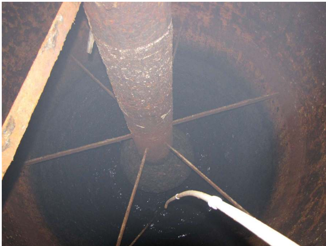
Sedimentation tank - interior
