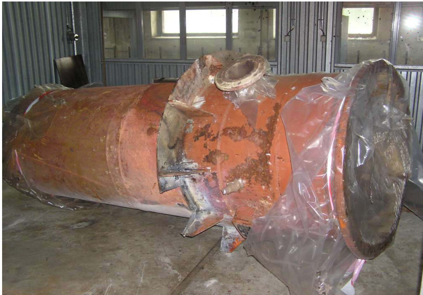
Heater before dismantling
