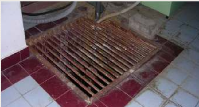
Common Pit (for contaminated effluent )
