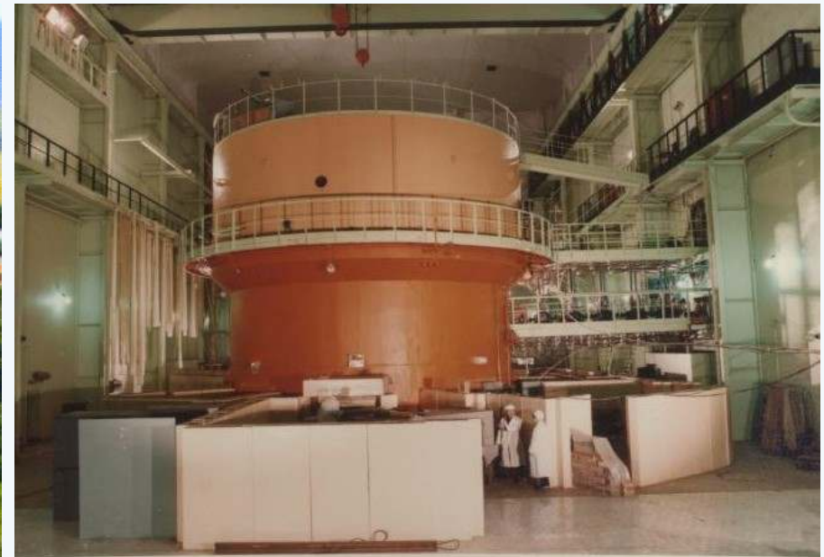
HWRR Reactor Hall & Reactor Block
