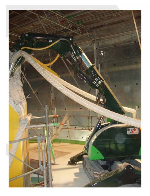
Demolishing by means of a Brokk demolition robot with local dust exhaustion
