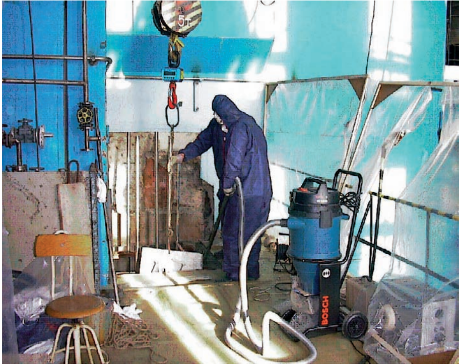
FIG. 5. Decontamination activities during refurbishment of the SRR's spent fuel pool.
