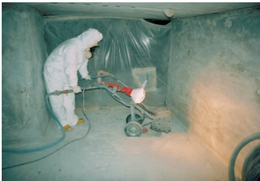
FIG. 10. Decontamination of a floor using a scabber, JPDR decommissioning project.
