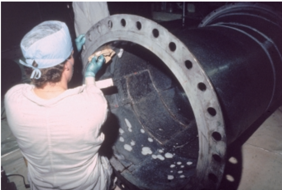
FIG. 6. Hand scrubbing during the decommissioning of Gentilly-1, Canada.
