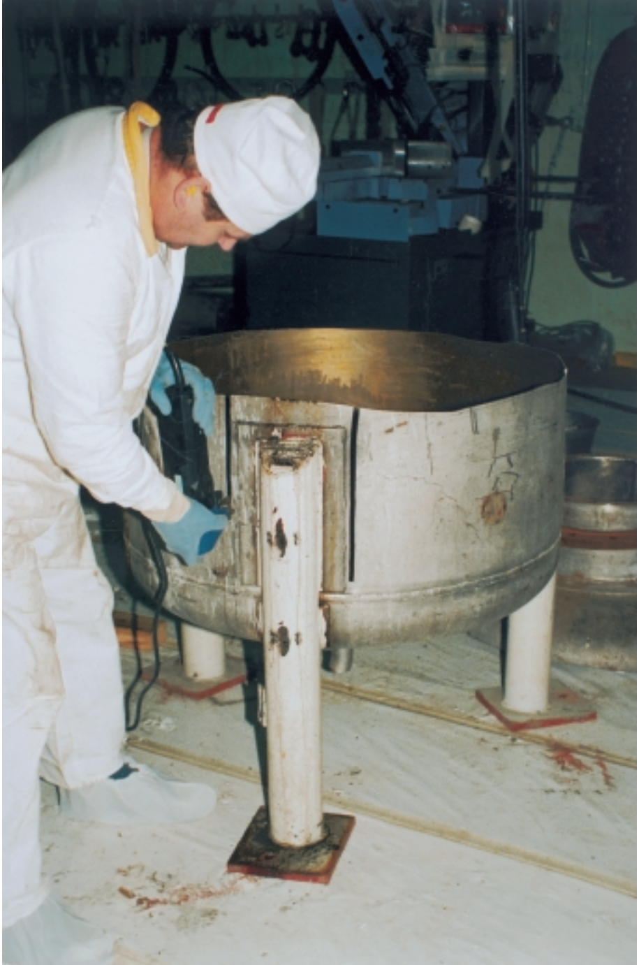
FIG. 16. Nibbler cutting thin plates, BR3 decommissioning project.
