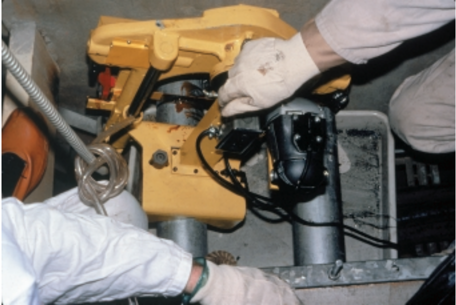
FIG. 19. Guillotine saw in use at Gentilly-1, Canada.
