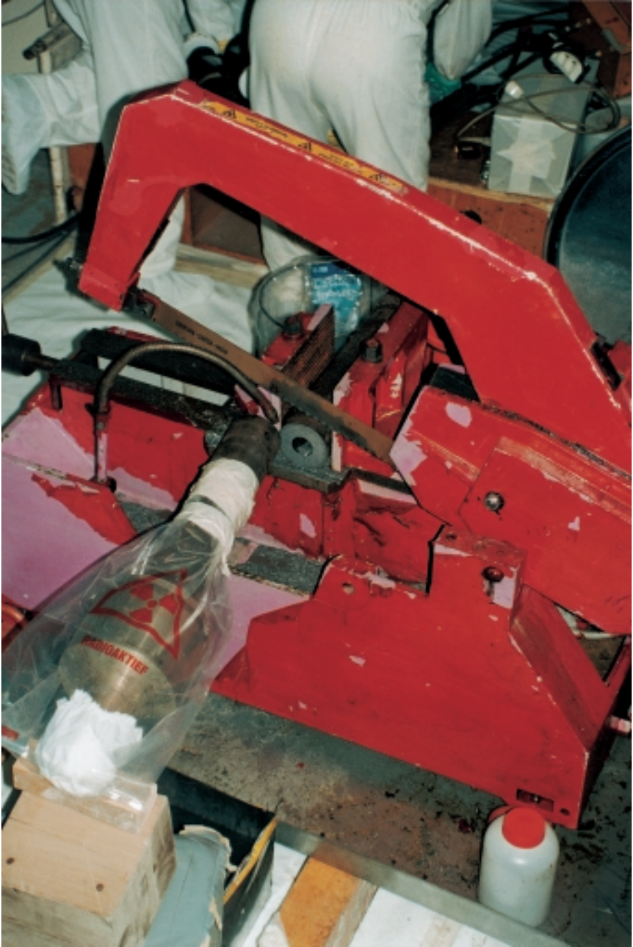
FIG. 18. Reciprocating saw in use at the BR3 decommissioning project.
