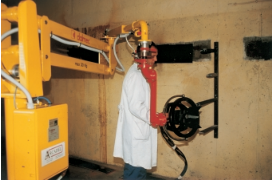
FIG. 14. Cutting pipes using hydraulic shears mounted on a balancer to reduce the physical load on operators.
