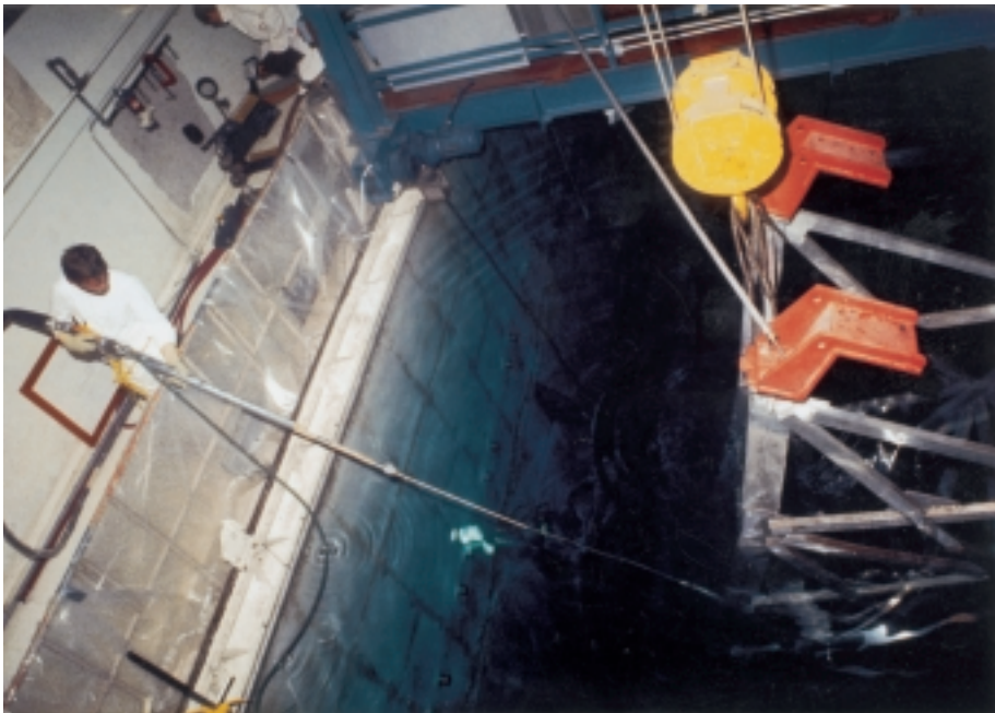
FIG. 8. Structural steel being decontaminated under water using a hydrolaser lance at Gentilly-1, Canada.
