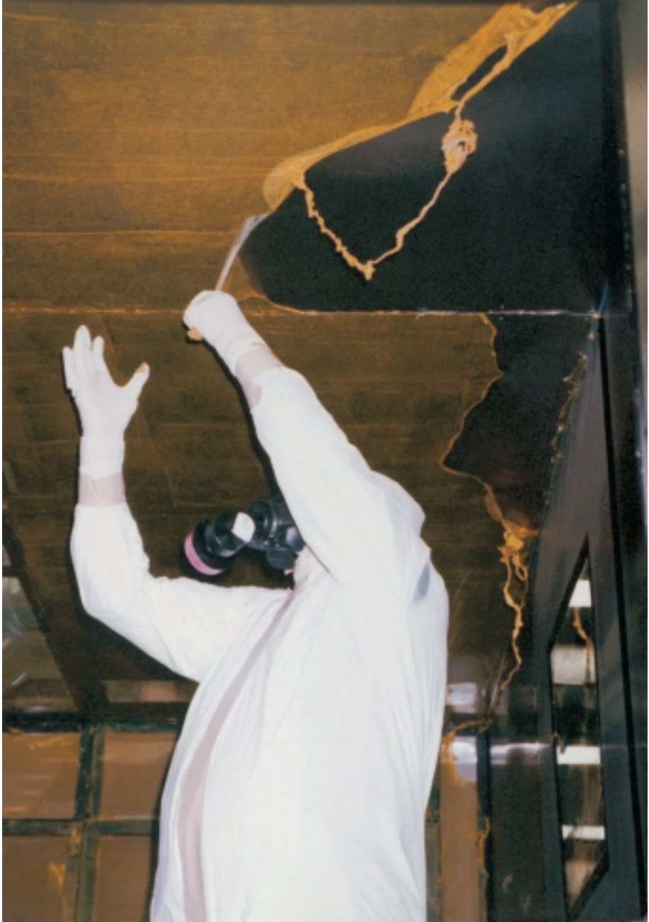
FIG. 7. Removal of strippable coating to decontaminate the glovebox size reduction containment. Courtesy Argonne National Laboratory, managed and operated by the University of Chicago for the US Department of Energy under contract No. W-31-109-ENG-38.
