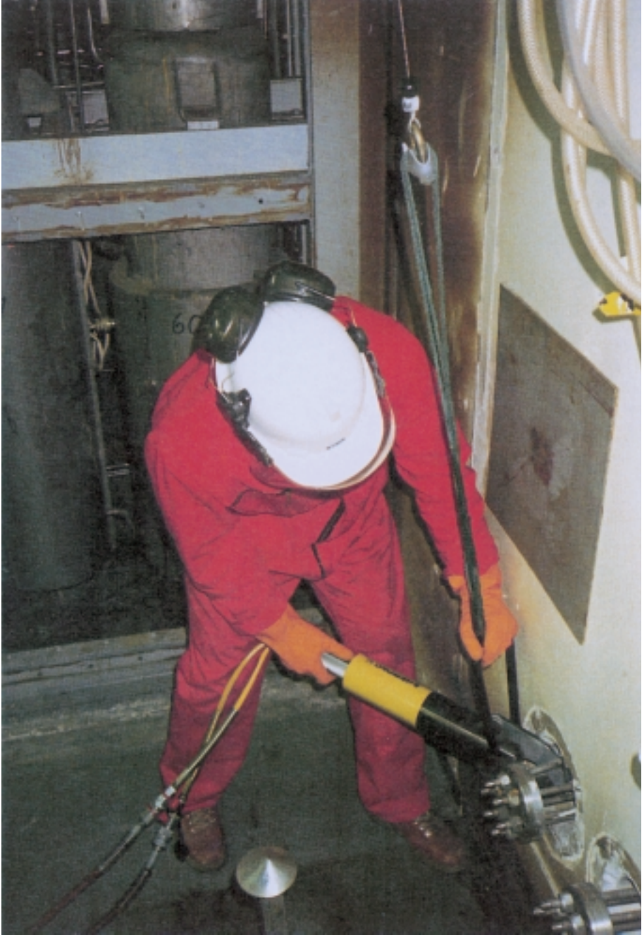
FIG. 13. Cutting with a hydraulic shear, Kjeller reprocessing plant, Norway.
