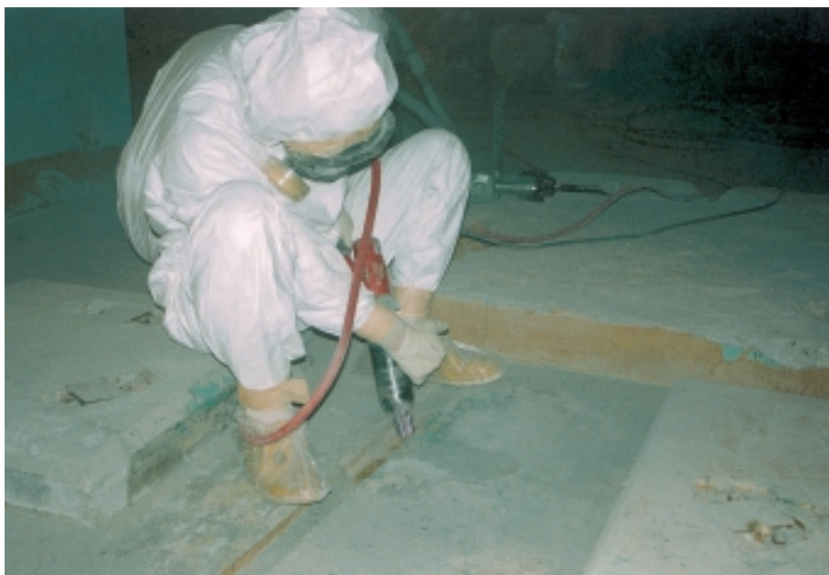
FIG. 11. Decontamination of a floor using a needle gun, JPDR decommissioning project.
