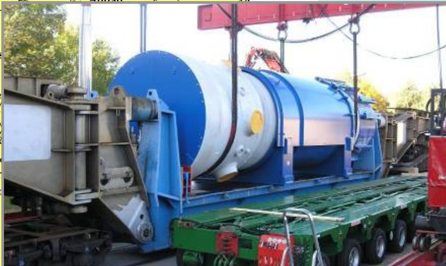
Transport of the Reactor Vessel
