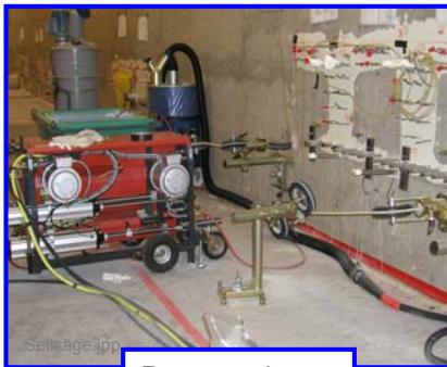
Rope saw in use
