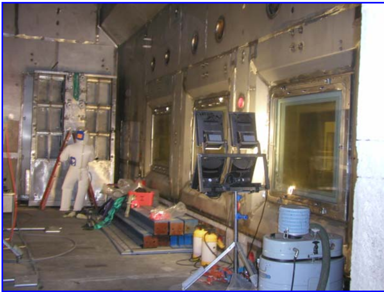
Mechanical dismantling cell: Prior to and after removal of the stainless steel liner
