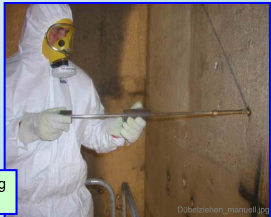
Drilling out of dowels
