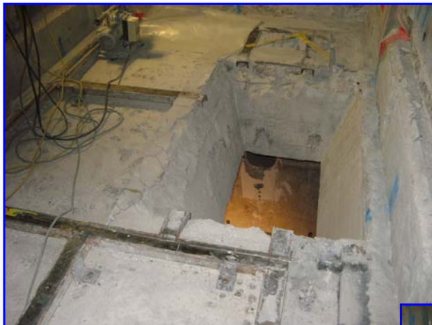
Mortising of concrete screed below the floor liner
