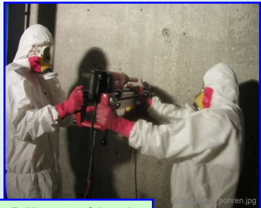
Drilling out of dowels
