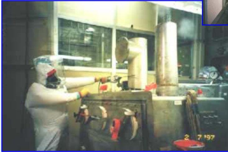
Dismantling of the Pu evaporator box in cell VIII using a compass saw
