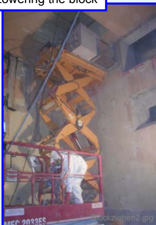
Lowering the block
