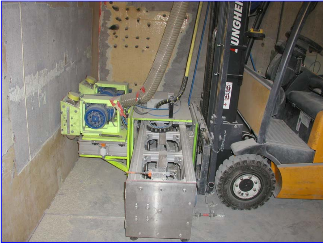
Forklift with attached shaver
