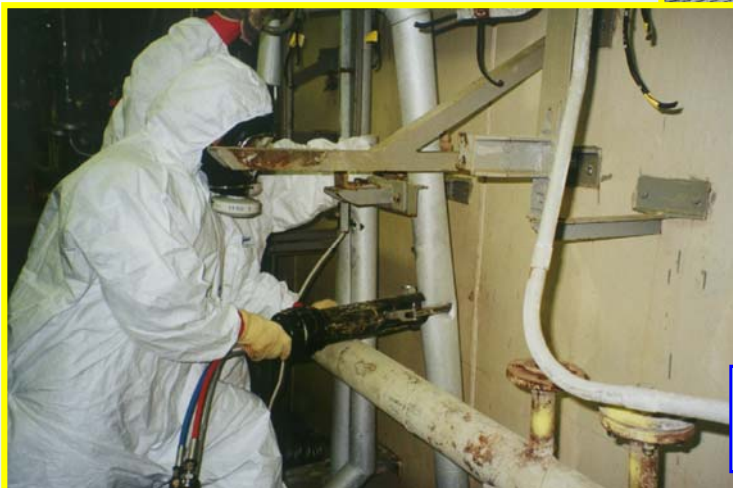
Cutting of pipelines by means of hydraulic shear
