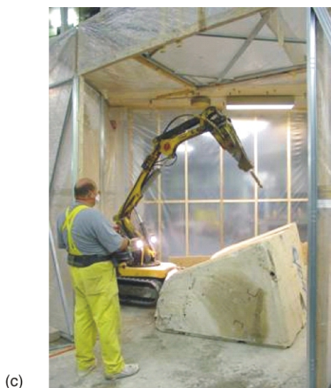
Figure 15. Dismantling the outer part of the activated zone
