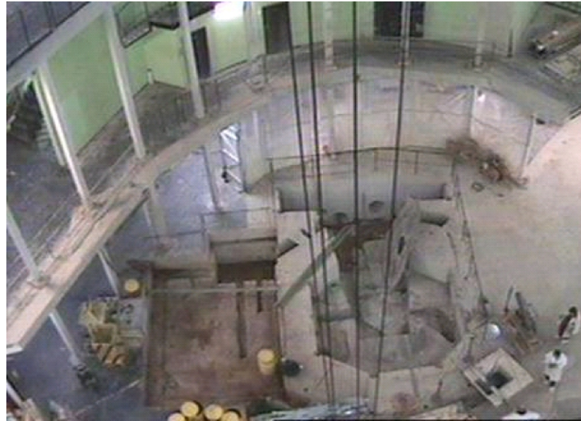
Figure 17. Removing of the primary tubing embedded within the foundations of the biological shield
