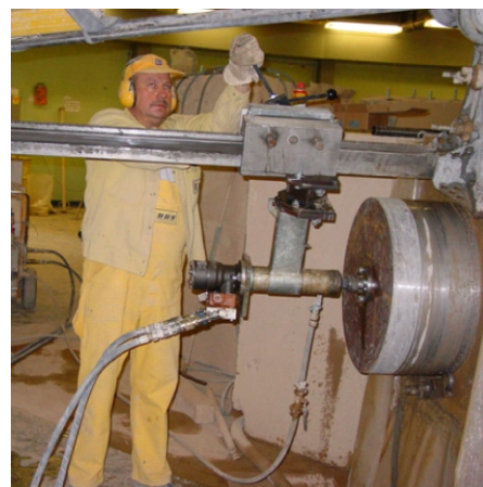
Figure 12. Core-drilling along beam tubes
