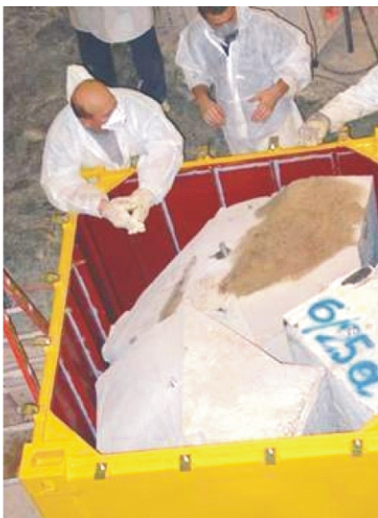
Figure 16. Dismantling the activated zone (a) Determination of cutting edges; (b) Dissecting in progress; (c) Storing the blocks
