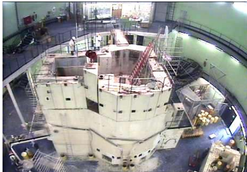
Block cutting at the upper shield
