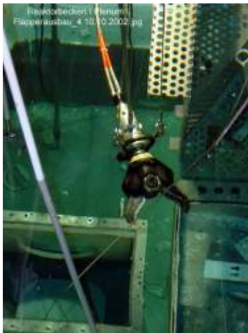
Under water cutting with hydraulic pliers
