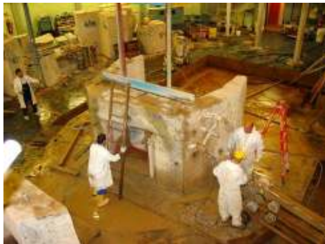
Dismantling at the activated zone
