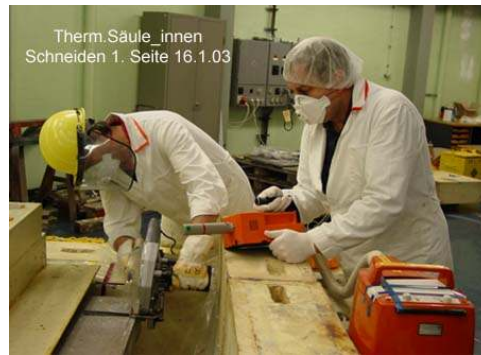
Removing and opening the „inner“ thermal column to recover the graphite rods for further heat treatment at the Hot Cells
