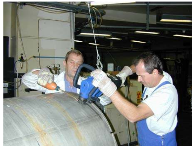
Opening of the inactive secondary side of a heat exchanger unit
