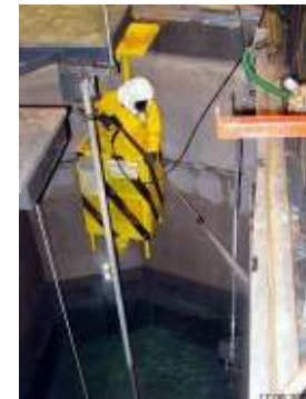
Cleaning the surface of the pool liner
