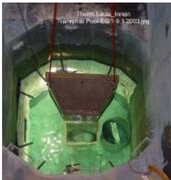
Removing and opening the „inner“ thermal column to recover the graphite rods for further heat treatment at the Hot Cells
