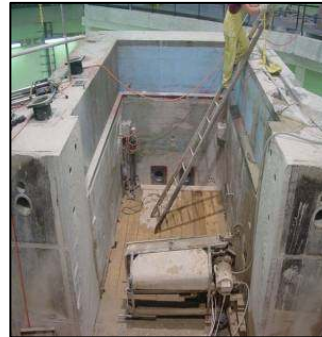
Application of diamond wire cutting saw
