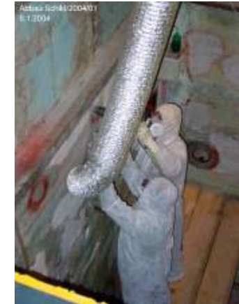
Removing contaminations from concrete structures
