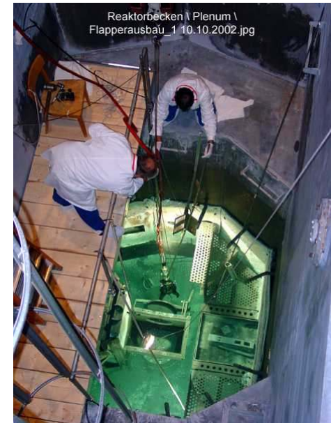
View of the ASTRA-core-area, decommissioning in progress
