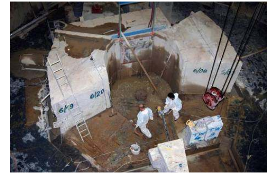
Block cutting at the lower shield area
