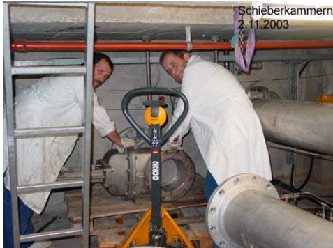
Dismantling primary circuit components in the valve pit within the reactor building
