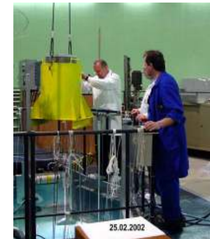
Transfer of activated parts to the Hot Cells for further dismantling
