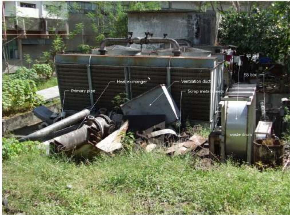
View of the Temporary Waste Store. Note the Cooling Tower in the background.
