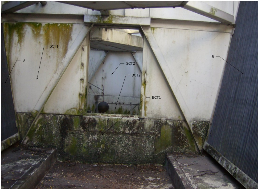
View inside the Cooling Tower. See Component List for labels.
