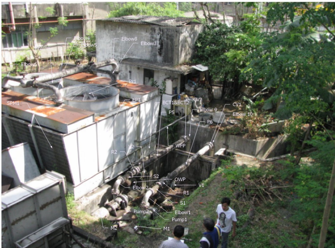
View of the south end of the Cooling Tower. See Component List for labels.
