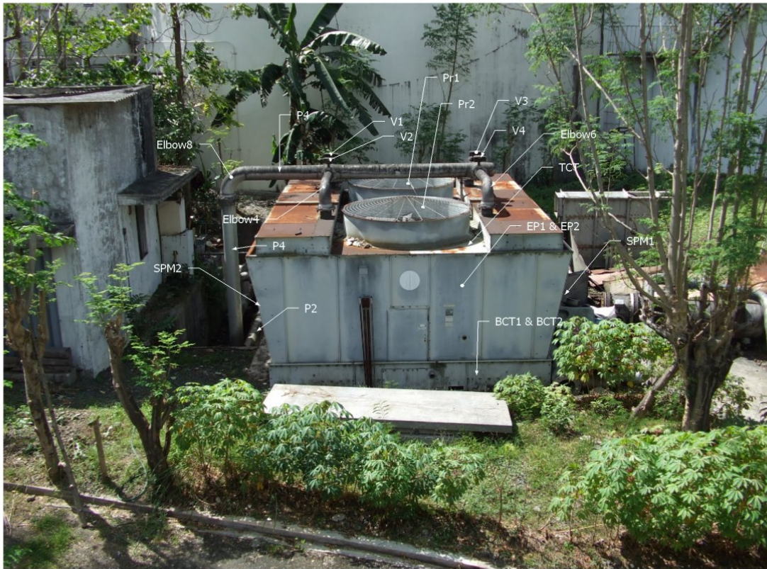
View of the north end of the Cooling Tower. See Component List for labels.
