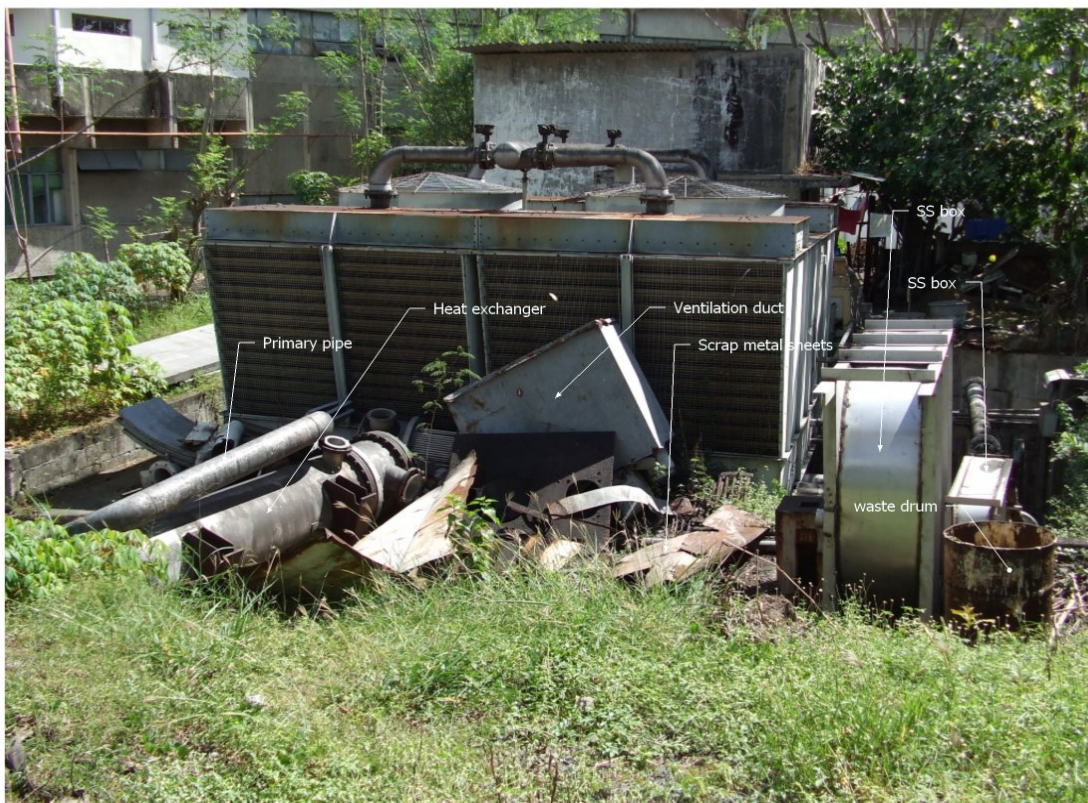
Another view of the Temporary Waste Store.
