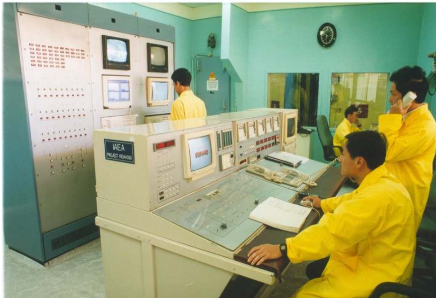
The control room of the DNRR
