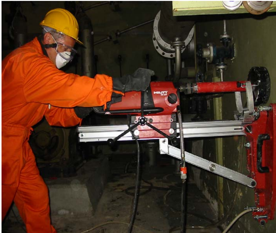
Figure no. 4.2 Diamond drill equipment for concrete core extraction - DD200
