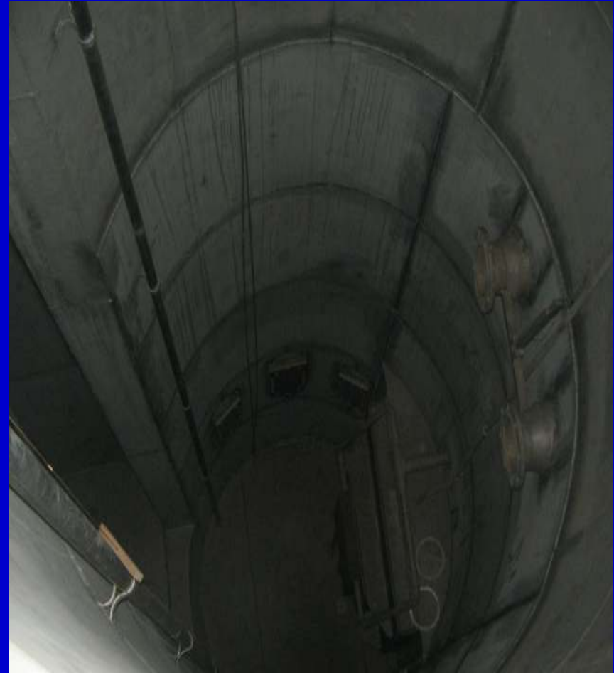
High power section
