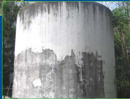
Raw Water tank (RG-10)
