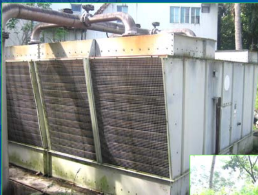
Cooling Tower (RG-11)
