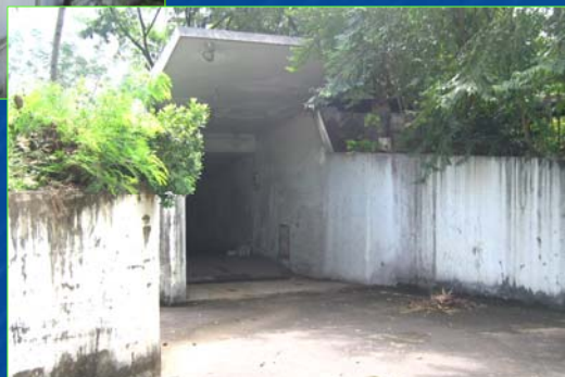
Truck Entrance (RB-3)
