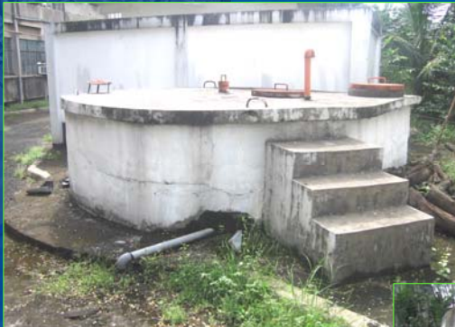
Diesel Fuel Tank (RG-9)
