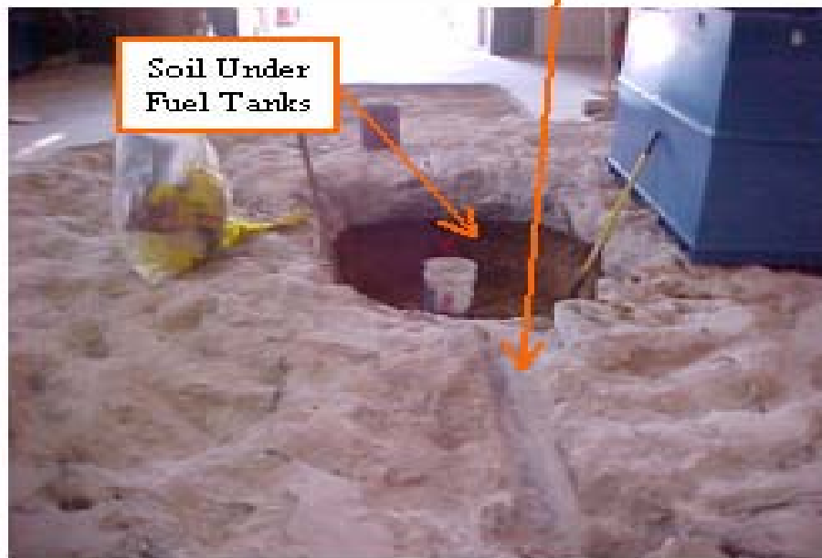
Figure 54. Activated Floor/Soil Removal
