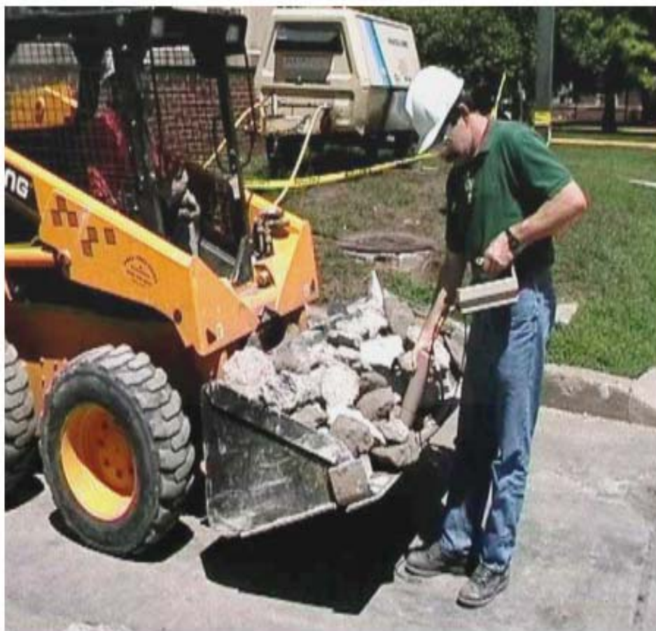
Figure 38. Waste Survey Prior to Disposal
