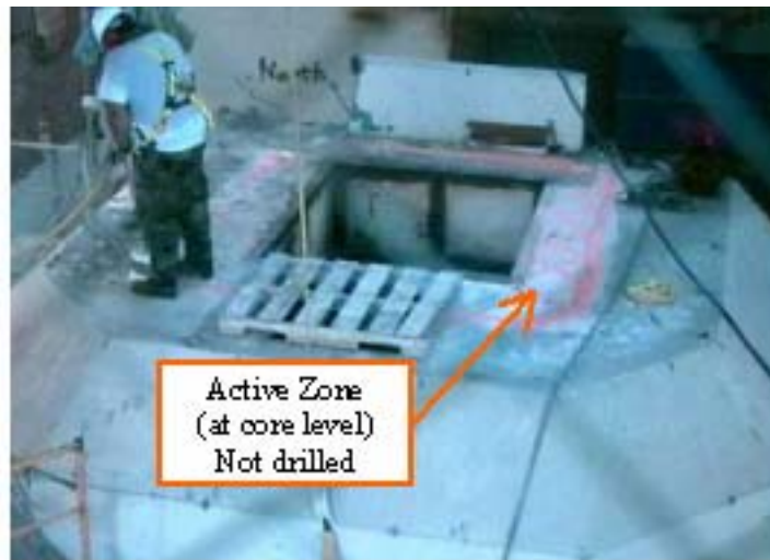
Figure 34. Drilling – 20 minutes per hole
