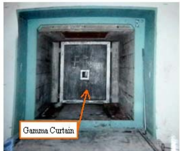
Figure 15. Graphite Removal Completed
