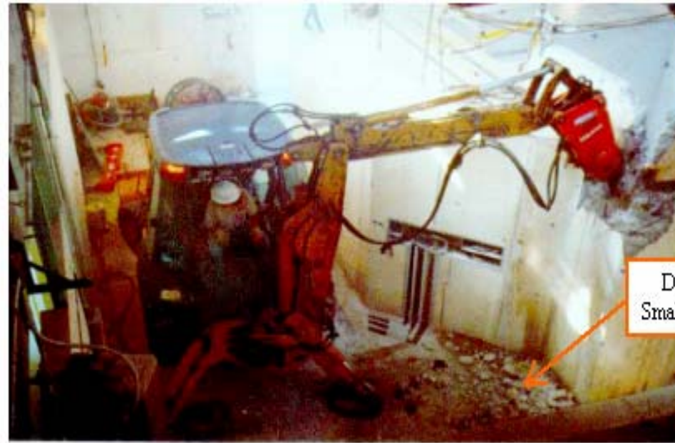
Figure 32. Day 1 – Jack-hammering Starts
