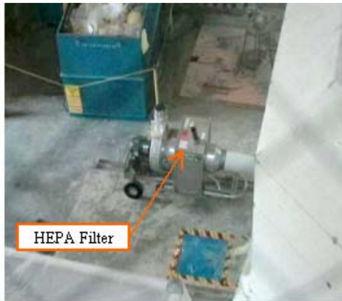
Figure 24. HEPA Filter Set-up
