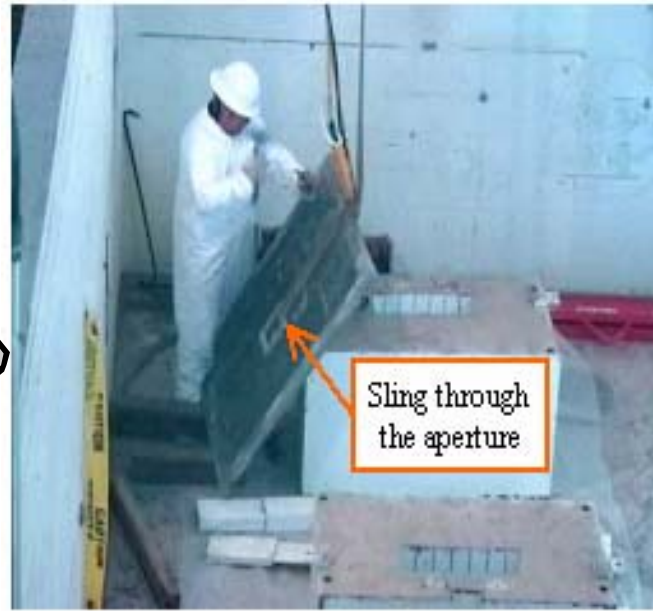
Figure 16. Aluminium Frame Removal
