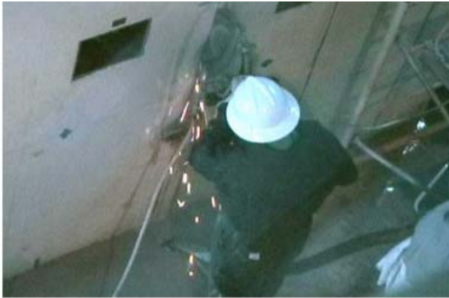
Figure 30. Scoring the Concrete
