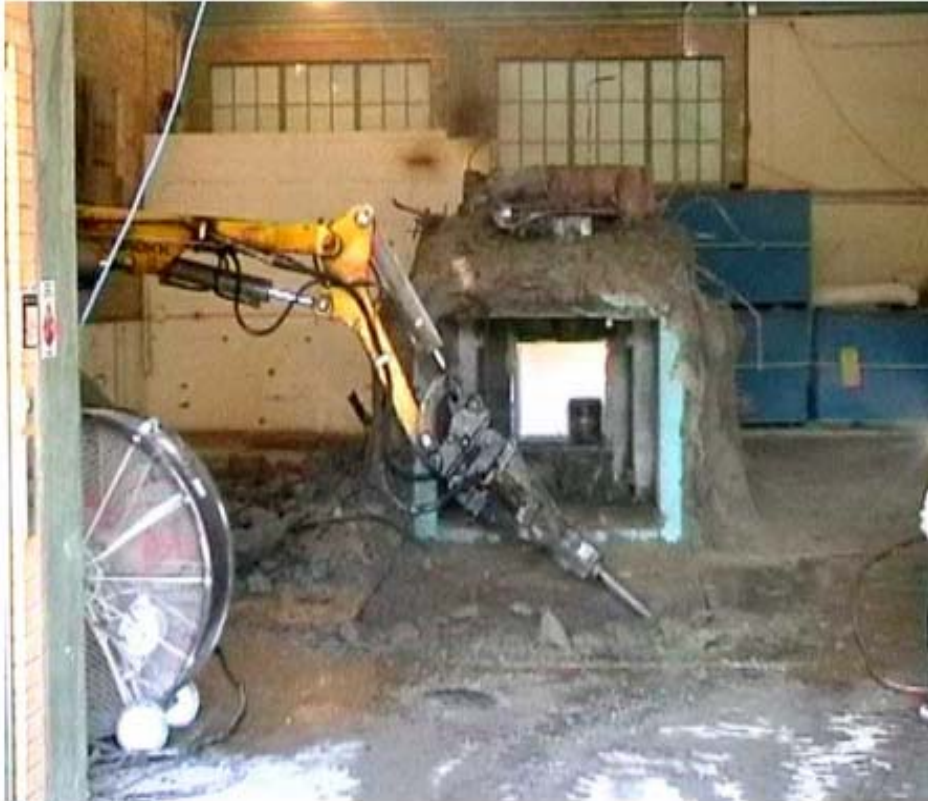
Figure 44. Day 4 (PM) – Floor Levelling
