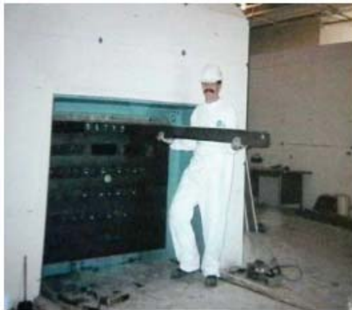
Figure 12. Graphite Removal by Hand
