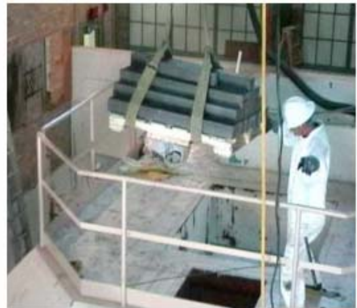
Figure 13. Graphite Removal by Crane
