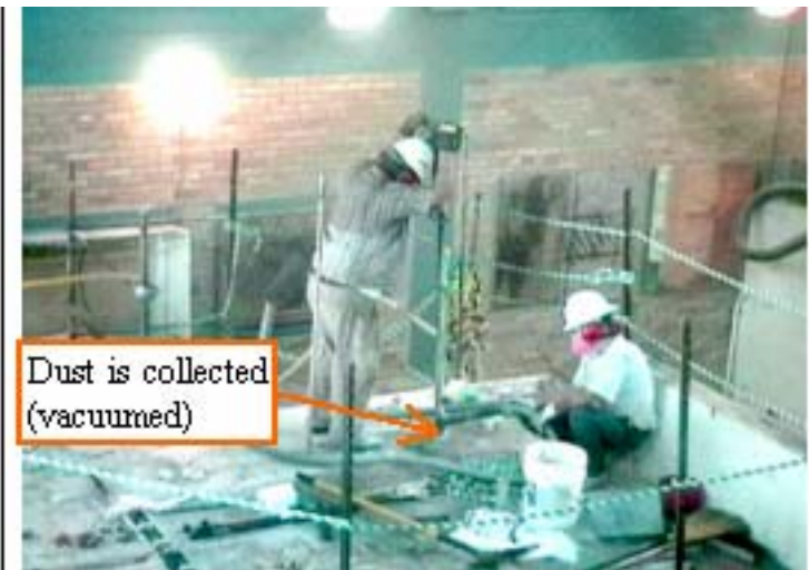
Figure 35. Drilling and Vacuuming
