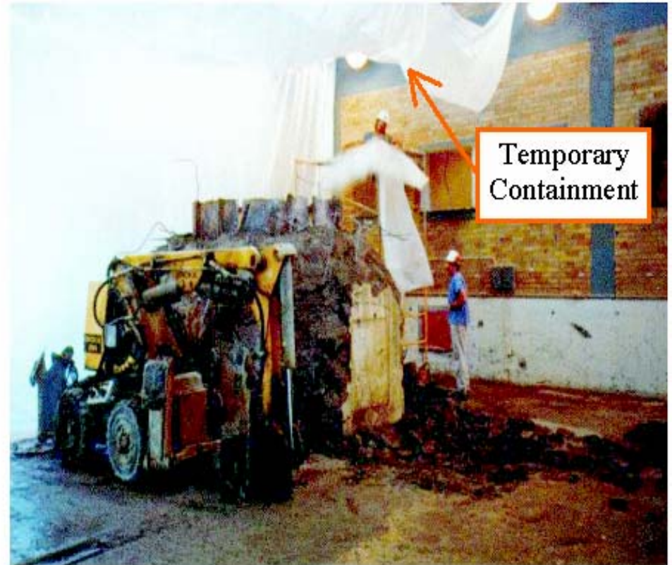
Figure 45. Day 4 – Containment Set-up
