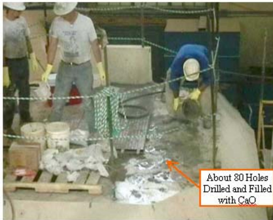
Figure 36. Holes being filled with CaO
