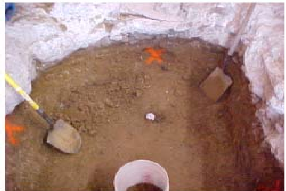
Figure 55. Activated Zone Excavated
