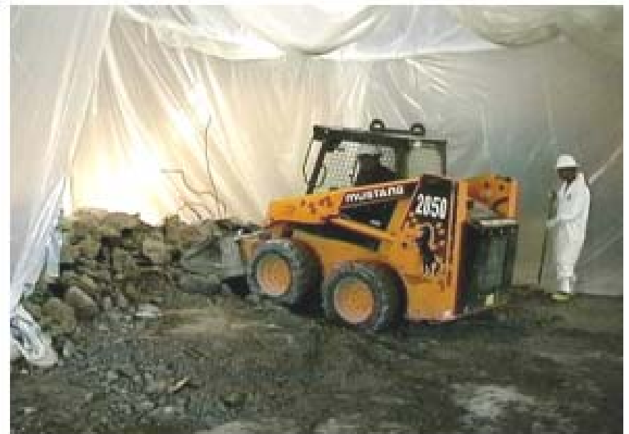
Figure 49. Day 5 – Active Waste Handling
