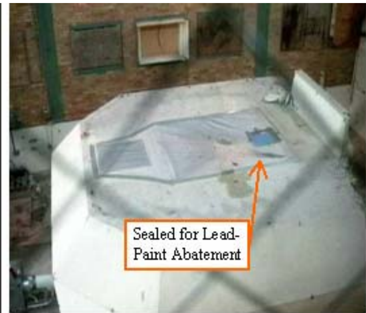
Figure 25. Paint Removal in Progress
