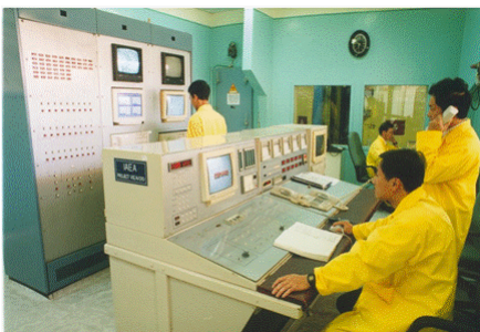
The control room of the DNRR
