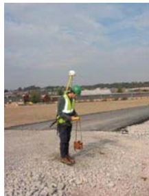
Work in progress measurement
