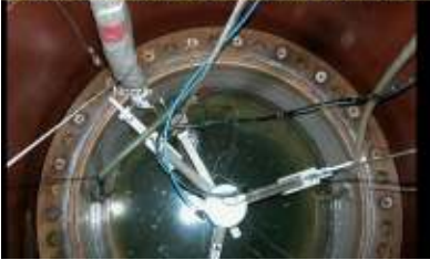
Remote controlled AWJ for cutting RPV and internals
