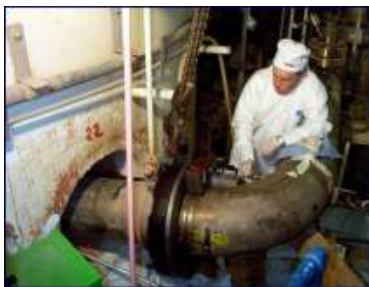
Orbital cutter to dismantle primary piping
