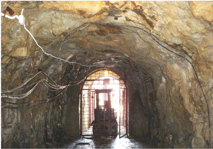
Entrance of Access Tunnel (looking out of the tunnel)
