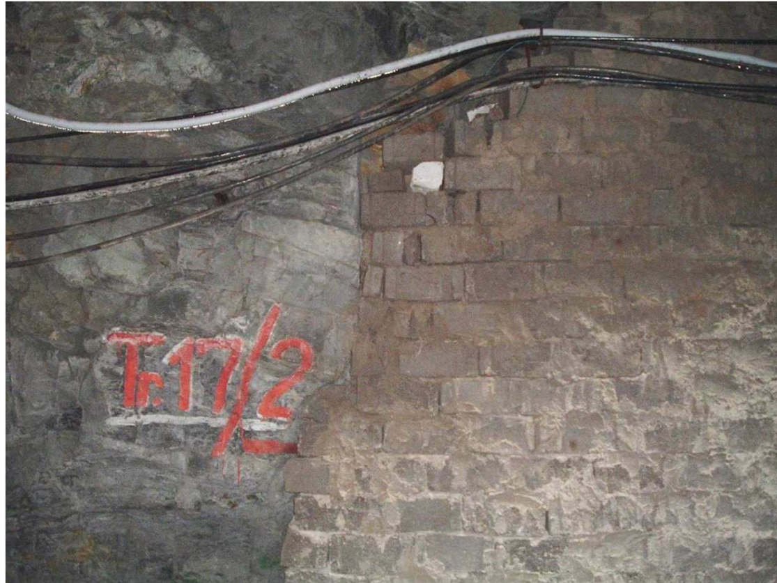
View of the Block Wall Sealing Disposal Gallery 17/2
