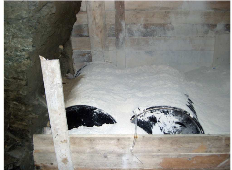
220 Litre Drums showing the Bentonite Backfilling and Wooden Shuttering
