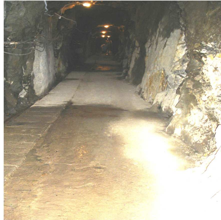
Access Tunnel with Covered Drainage Channel
