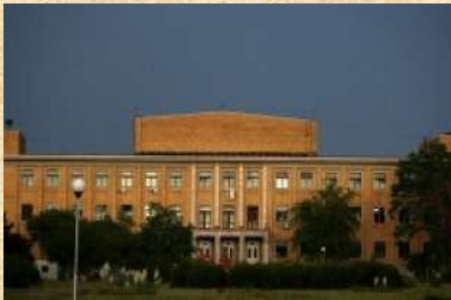
Fig. 1 VVR-S Nuclear Research Reactor
