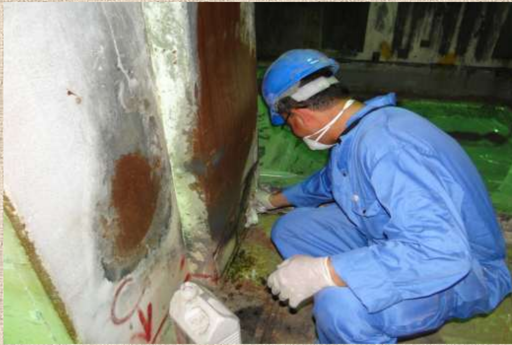
Decontamination of hot cell A
