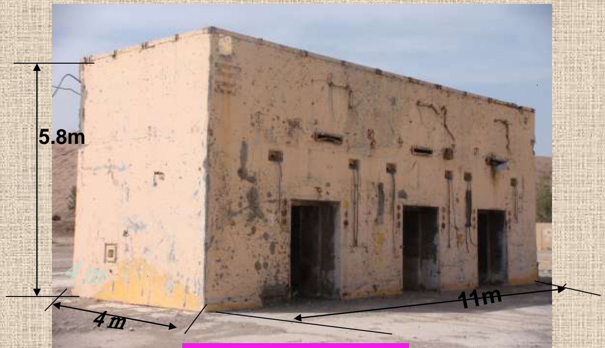
Three concrete hot cells
