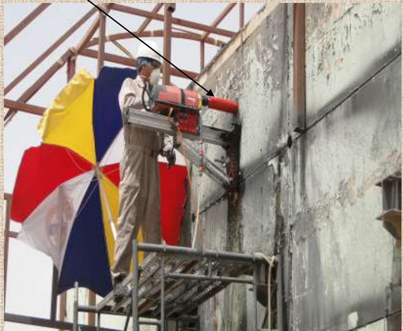
DIAMONDCORING BY DD 500
