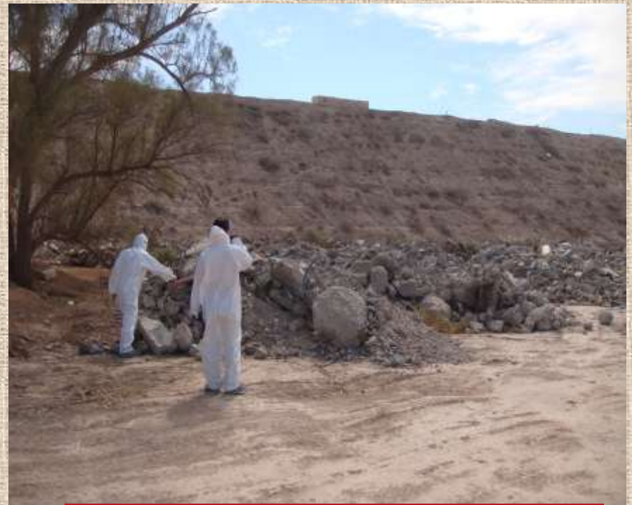
Clean rubble & concrete area
