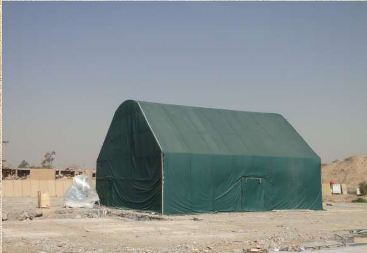
Tent to isolate hot cells during decontamination
