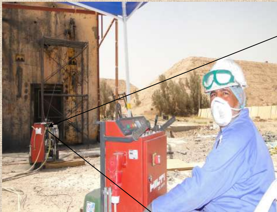
DIAMONDCORING BY DD 500
