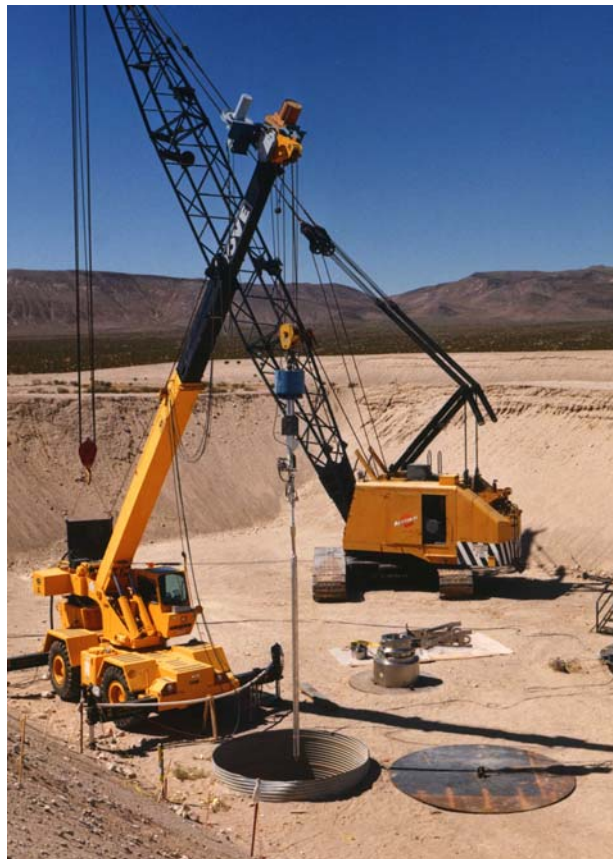
Figure 5-8: Historic, Remote Disposal of Reactor Fuel Rods in 36-m Deep, 3-m in Diameter GCD Boreholes (Spend Nuclear Fuel was Removed Prior to Disposal)
