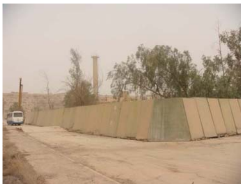
Figure 7-1: Perimeter Fence Installed for LAMA Phase 1 Dismantlement
