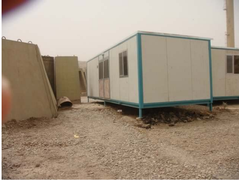
Figure 7-2: One of the Portable Buildings Installed for the LAMA Stage 1 Work
