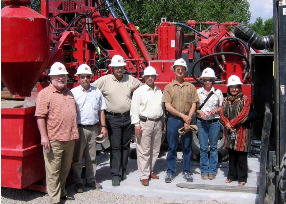
Figure 4-8: MoENV, RPC and DOS Representatives Observing the Drilling of a Monitoring Well at Water Development Corporation's Field Office
