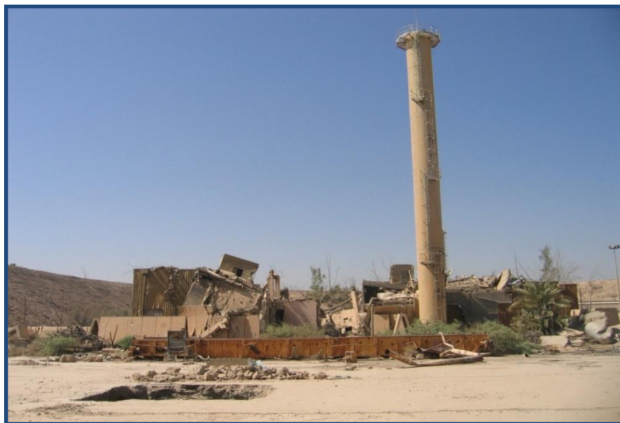
Fig. 2 Decommissioning of the Destroyed LAMA Facility
