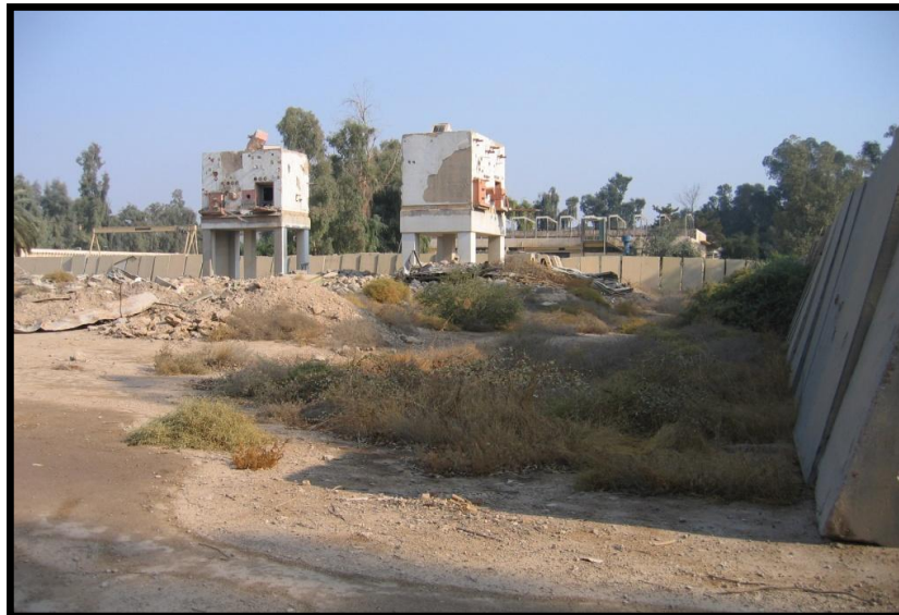
Fig.4 Decommissioning of Radioisotope production facility
