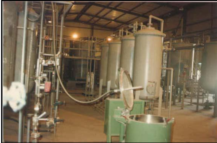
Fig. 3 Decommissioning of Geo Pilot Plant
