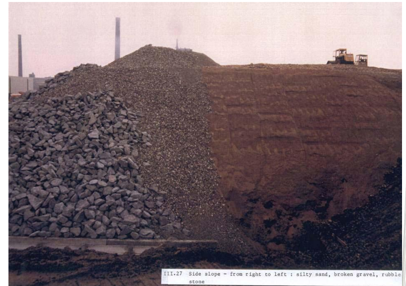
Side slope – silty sand, broken gravel, rubble stones
