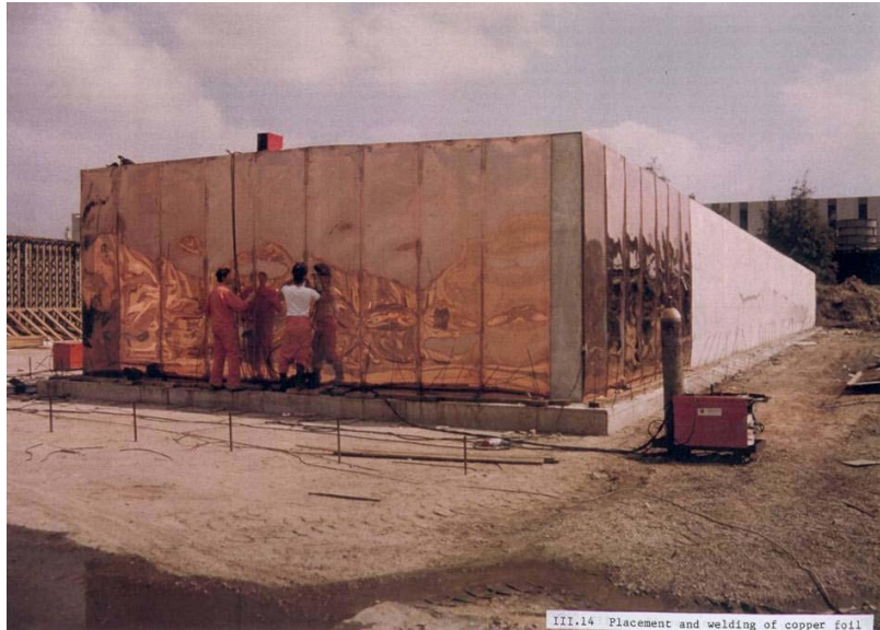
Welding of copper foil
