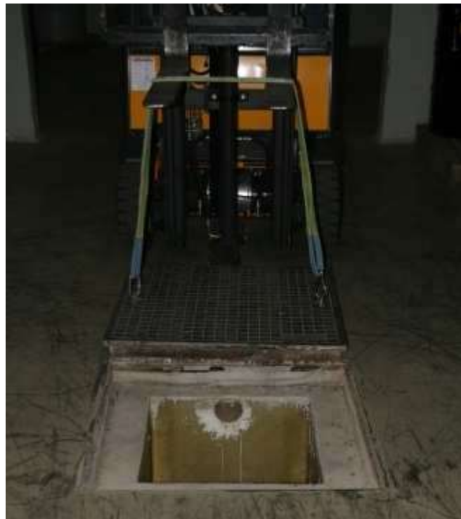
FIG. 13. System for collection and retention of liquids.
