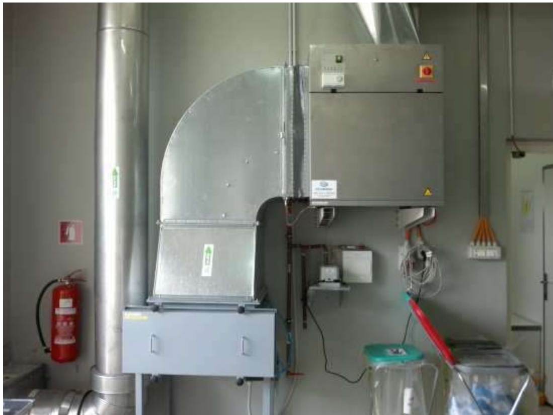
FIG. 17. Heating and moisture control system.
