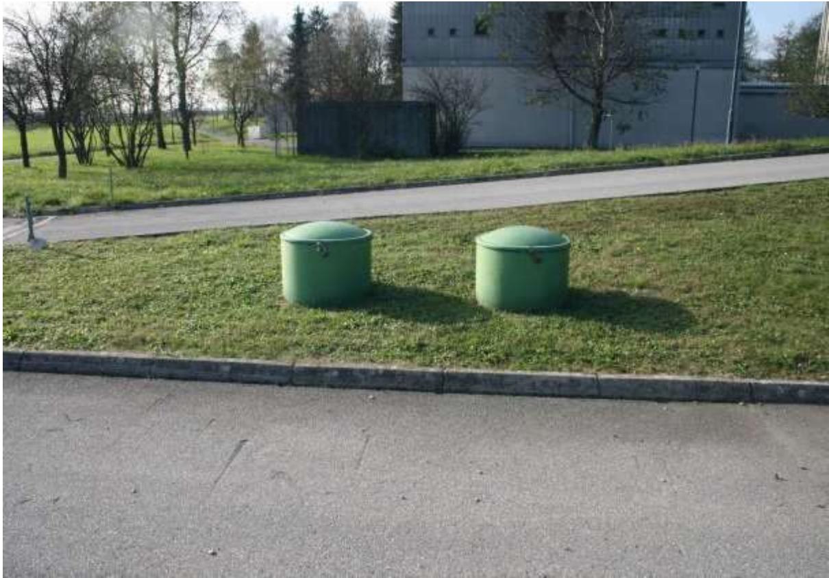
FIG. 14. System for collection and retention of liquids, outer part.
