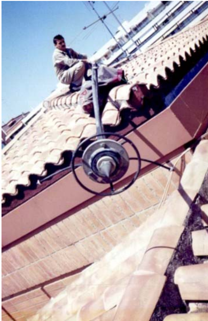
Figure 2. Removal of radioactive lightning rod headers.
