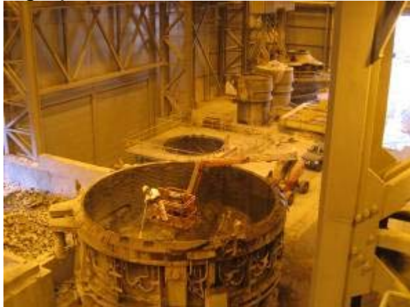
EAF preliminary cleaning with high pressure water.
