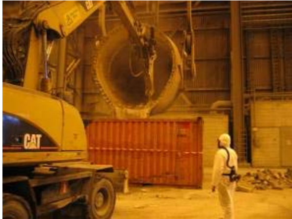
Ladle dismantling work at masonry work shop
