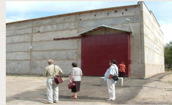
Concrete storage building
