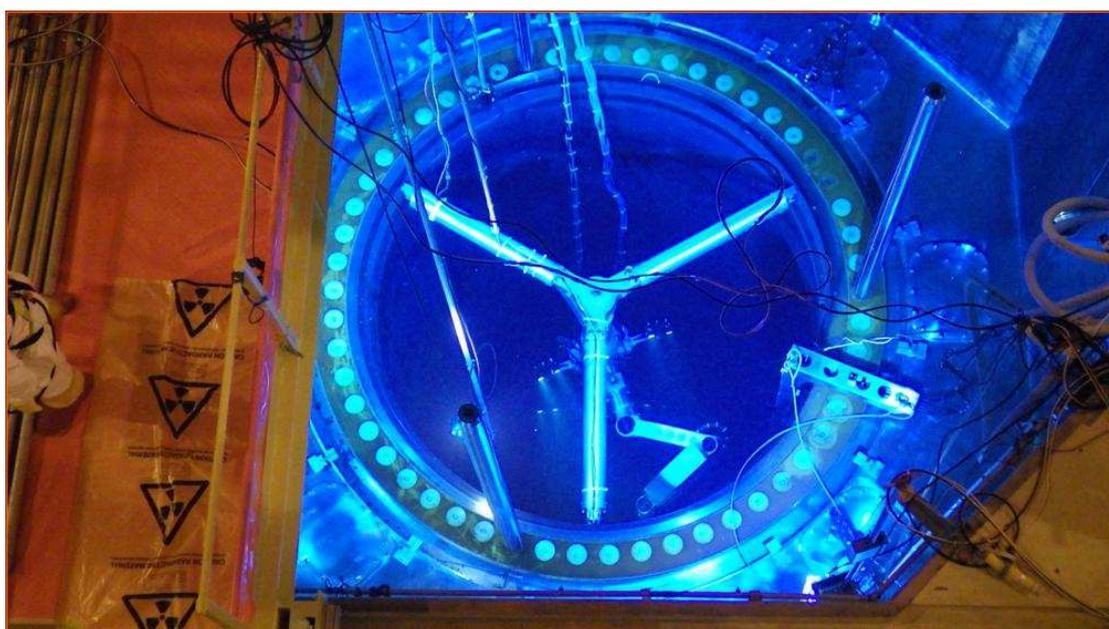
**Figure 7 – Photograph of reactor pressure vessel (RPV) at Sizewell B**
