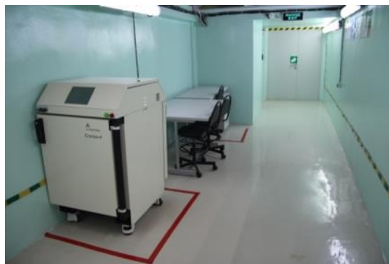
Place for waste sacks monitoring
