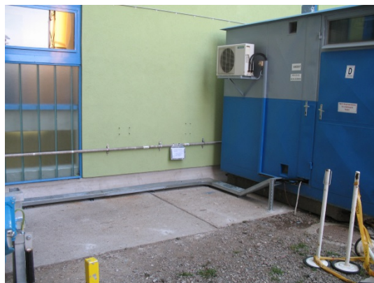
The temporary cable
