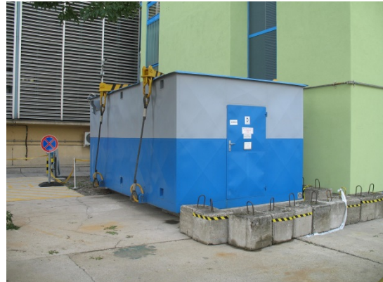
Container battery plant
