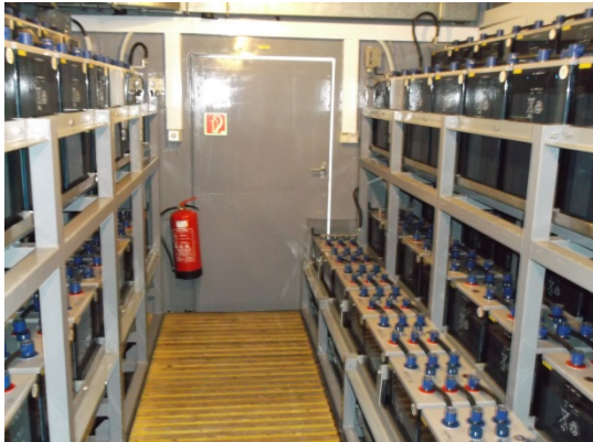
The interior of the battery plant
