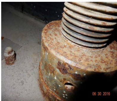
ARE system pipe fixed point anchor bolt
