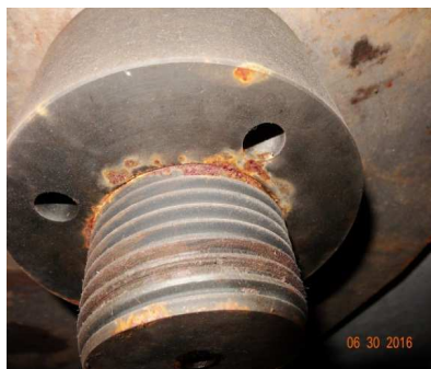
RIS system pipe support bolt
