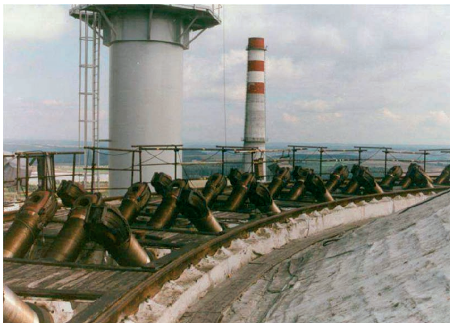
FIG. 5. Pre-stressing cable in a cylindrical wall — picture from the construction period (source: SUJB, Czech Republic, IRS meeting 2008).
