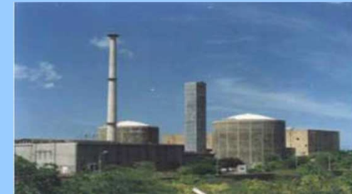
PHWR 1-170 MWe, 2-220 Mwe KALPAKKAM
