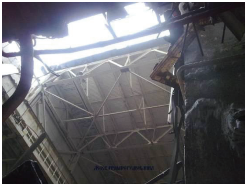
Damaged roof of the turbine hall of Unit 4 at the Chernobyl nuclear power plant (Photo Credit: State Nuclear Regulatory Inspectorate of Ukraine).
