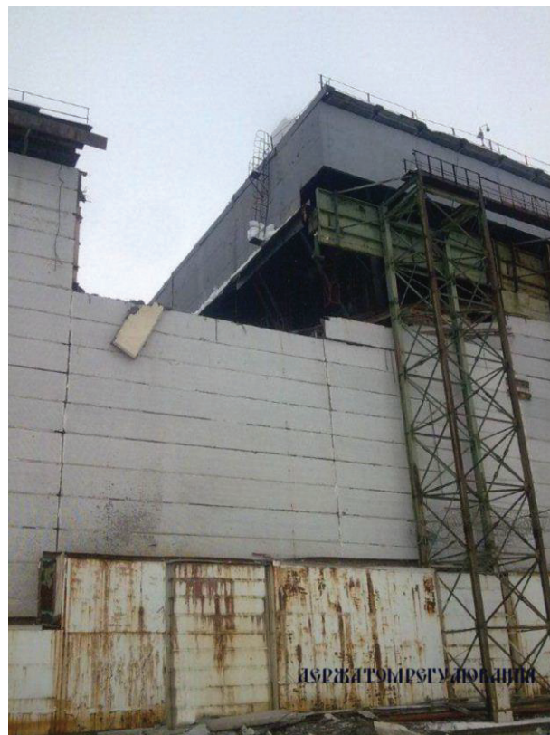
Damaged wall of turbine hall of Chernobyl NPP Unit 4 - view from waterside pump station (Photo Credit: State Nuclear Regulatory Inspectorate of Ukraine).
