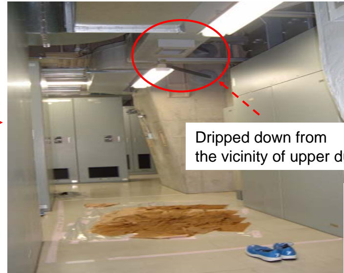
Reactor building mezzanine 3rd floor where leakage water dripped down (non controlled area)
