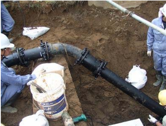
Status of restoration.
