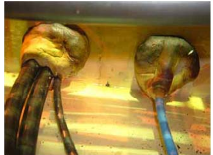
Cable for refueling machine (under floor)
