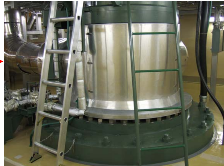
Residual Heat Removal Pump (B5F in the reactor building).
