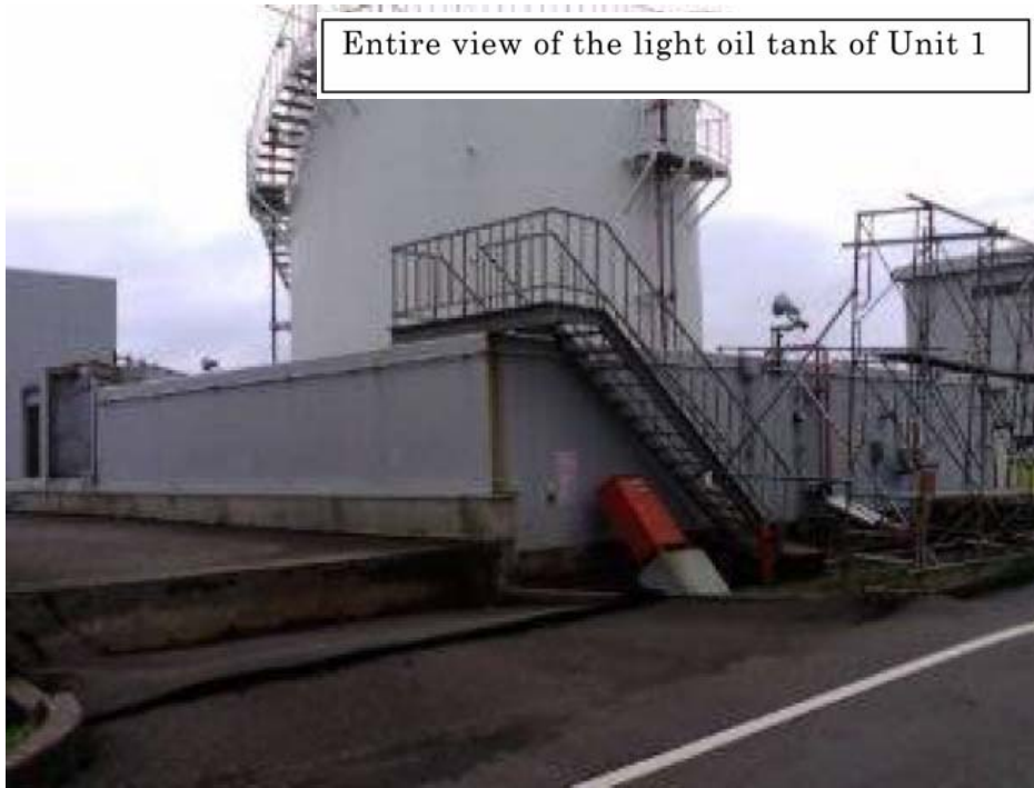
Entire view of the light oil tank
