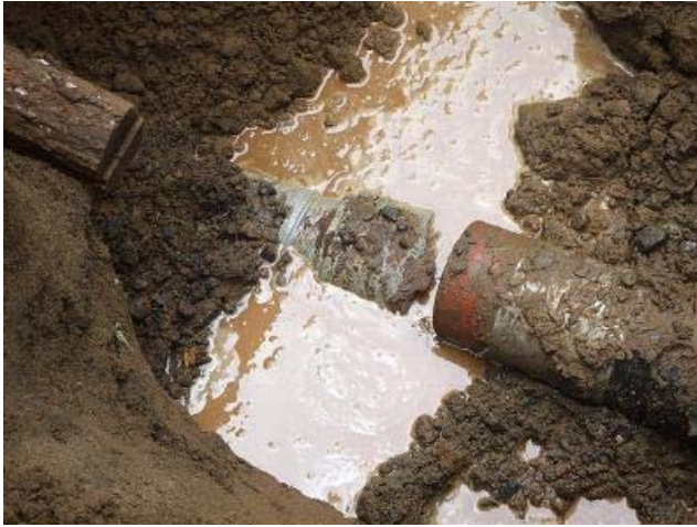
Status of damage.
