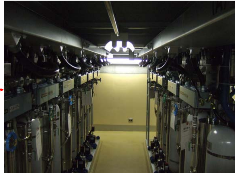
Residual Heat Removal Pump (B5F in the reactor building).
