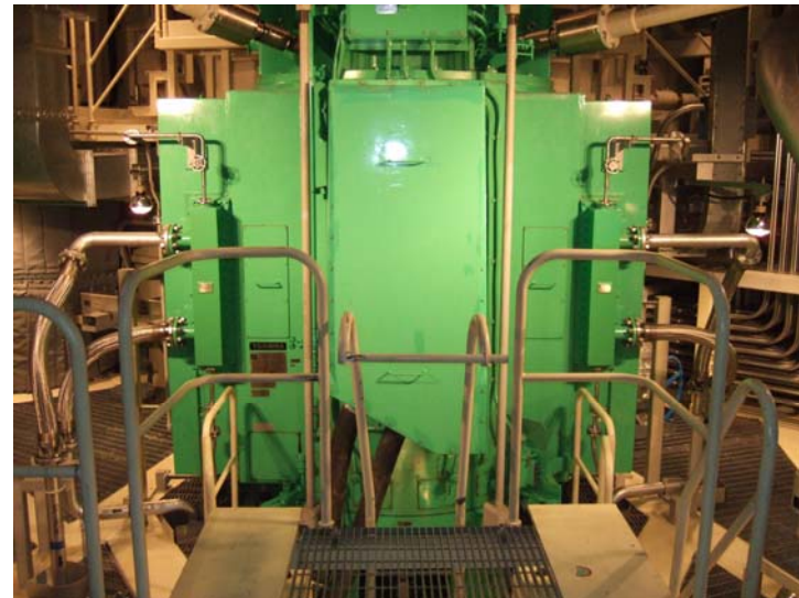
PLR pump (In the primary containment vessel).
