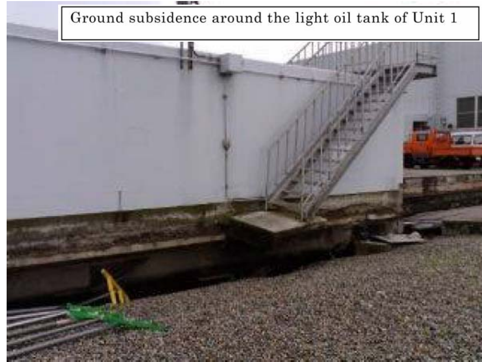
Ground subsidence around the light oil tank
